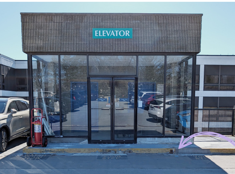
Glass-walled elevator entrance with a green "Elevator" sign above mounted on a concrete roof. A curb with yellow edges is in front of the elevator enclosure. It is flanked by parked cars and a fire extinguisher on the left. In the background is an office building under clear skies.
